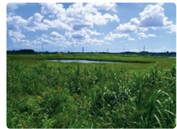
Shibakawa Daiichi Flood Control Reservoir
