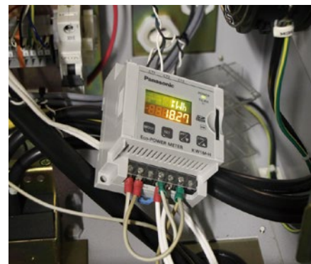
Streamlined electric power management sensor (being used to measure the electric power consumption of an NC lathe machine at the Hirosaki Plant)
