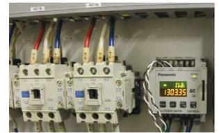
Streamlined electric power management sensor (Being used to measure the electric power consumption of the washing equipment at the Namioka Plant)
