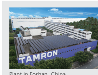
Plant in Foshan, China
